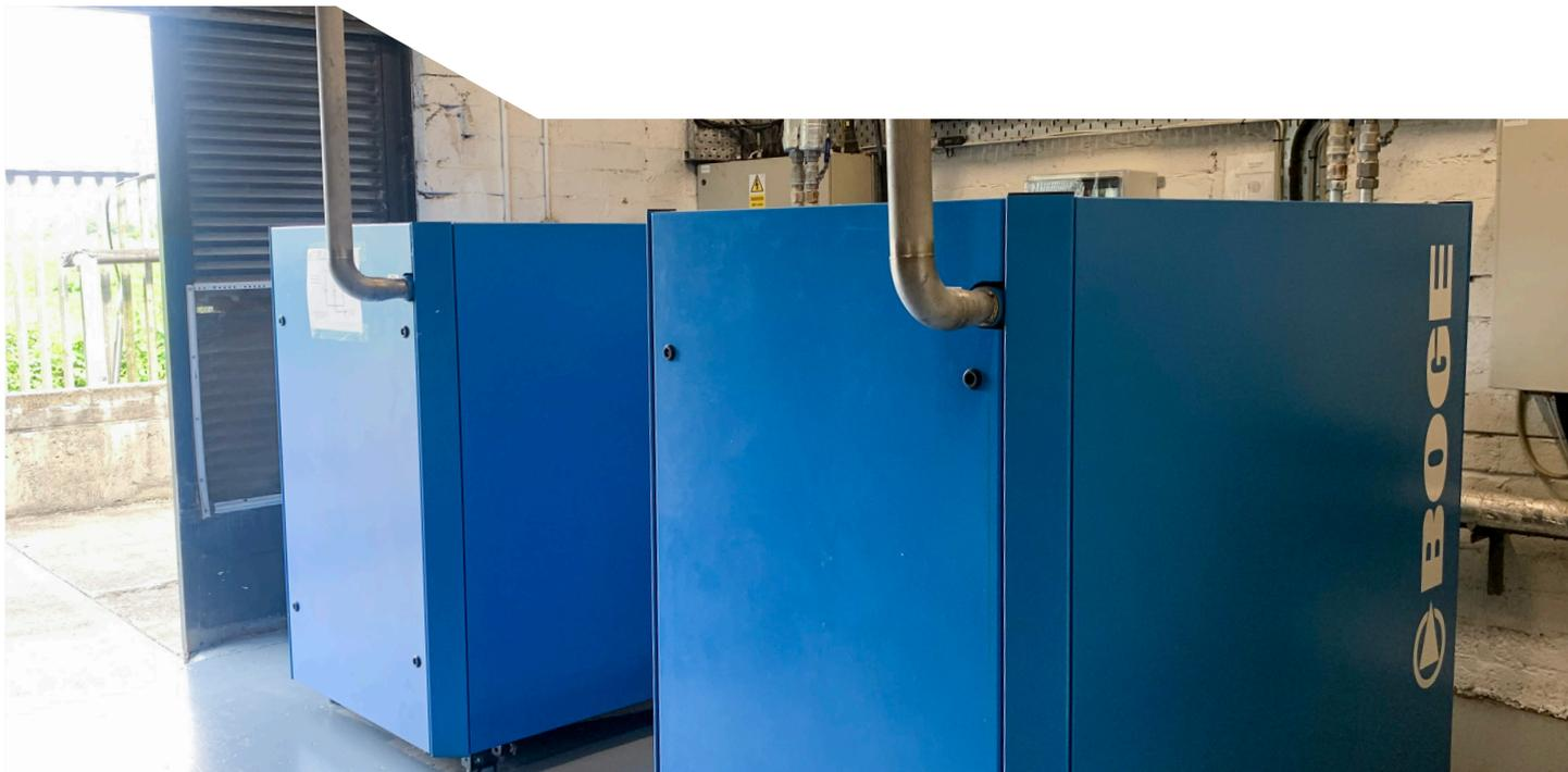
He continues, “We applied data loggers to the system to monitor its energy use. We were then able to estimate how much could be saved by replacing the existing 55 kW and 30 kW units with more modern compressors and adding heat exchangers. The customer agreed to our proposal.”
