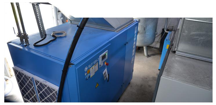
Installation took just two days and was completed during the Christmas break with no interruption to production. The old duty compressor has been retained as a standby, while the old standby will also be available for use.
